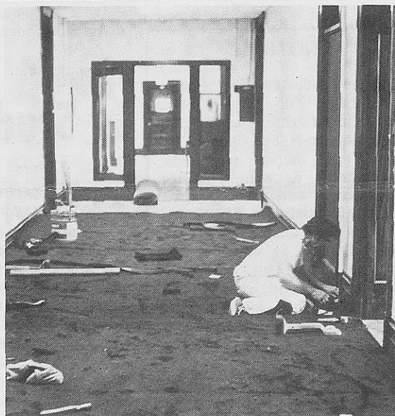
Renovation for Media Center continues on Second Floor of Ad. Building.
